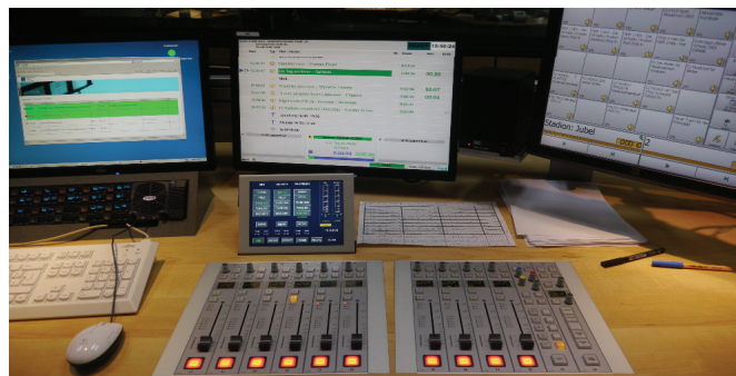
Key to the NDR upgrade was the requirement for all computer terminals to be instantly connected and switched with the data centre several floors below
